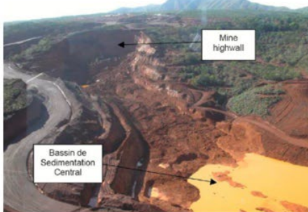
Photographs of 2006 highwall slope failure in Goro, New-Caledonia.
