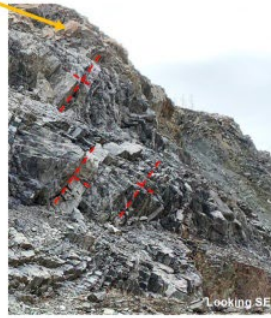
Discontinuities steeply dipping into the pit along with orthogonal set(s). Rockfall hazard mitigation included significant scaling, as well as fencing.
