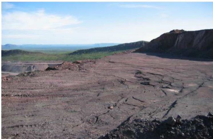
Bench with visible tension cracks indicating instability.
