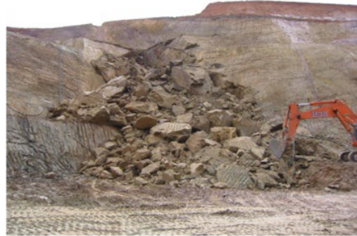
Wedge failure impacting spotter resulting in 1 fatality
