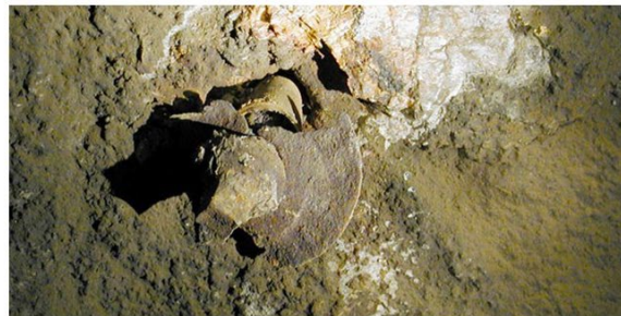
Poorly Installed Bolt
