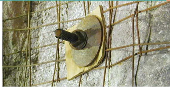
Well Installed Bolt
