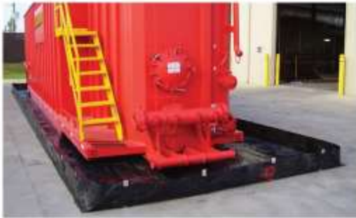
This is not adequate containment for this size of tank!
